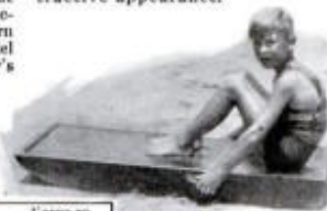
Fig. 2. The surf sled can be used in any sea not too dangerous for ordinary bathing. The rider holds himself by the handgrips or lies flat on the deck. In Fig. 3 is shown a slightly improved design.
