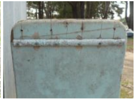
Nose with double reinforcements Photo courtesy Bryan Hayden
